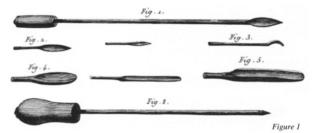
Figure 1 is the well-known picture of the woodwind makers tools from the *Encyclopédie ou dictionnaire raisonné des sciences, des arts et des métiers* by Diderot and d'Alembert (1751-1780). It shows pointed drills (fig. 1 and 2) as well as short reamers (fig. 4 and 5), more or less in the shape of a spoon (fig. 4). The tool of fig. 3 is probably a 'scraper', for widening a bore over a short distance, for instance close to the fingerholes.
